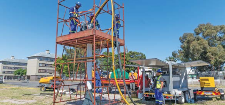
Ditching trenches for this one: City team members hard at work on the rehabilitation of 2 330 m of sewer pipe in Kewtown, Athlone. Thanks to the state-of-the-art 'cured-in-place piping' method, there is not a trench in sight.
